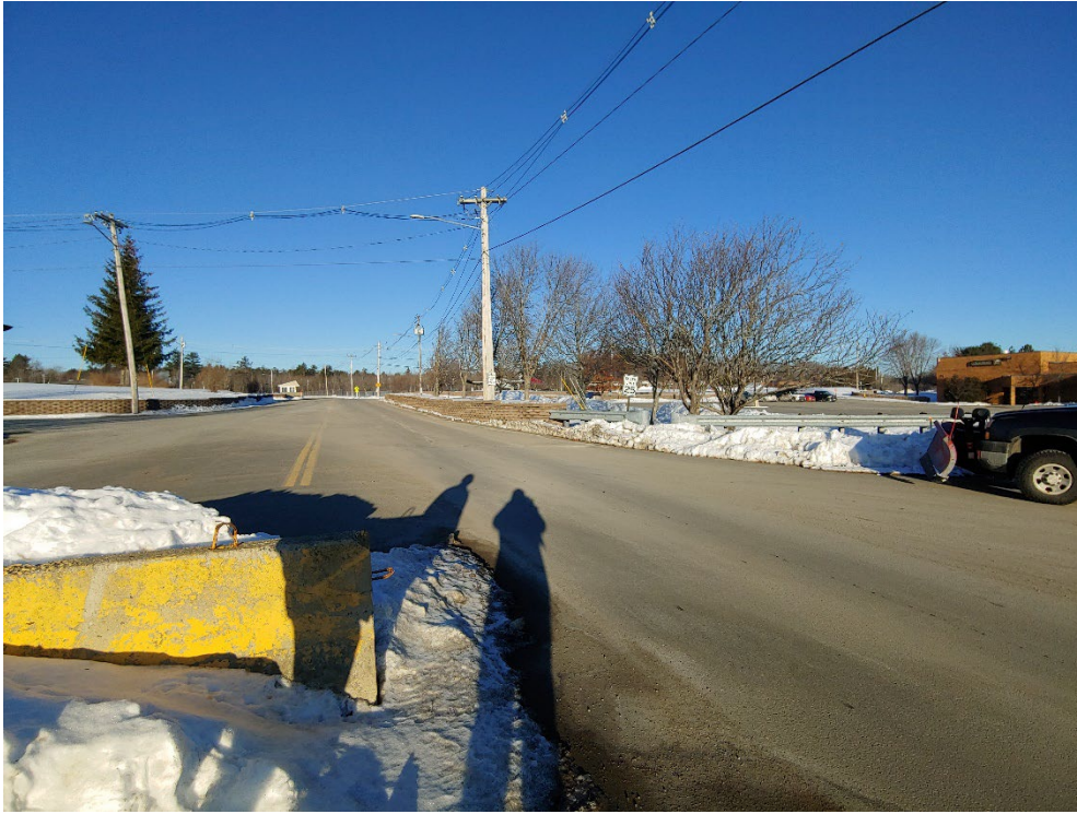
Project 2. Repair Main Entrance AT/FP (inside the gate) (FKNN162349): View on base from the main gate looking northwest down Maineiac Avenue. (Photo credit: L. Rivard, Tetra Tech, 1/11/2021.)
