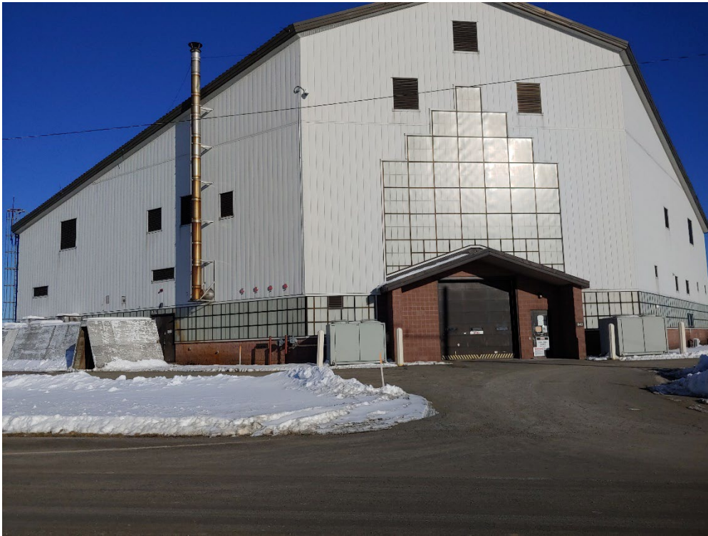
Project 8. Demolish B542 (FKNN252001): View of B542, looking north. (Photo credit: L. Rivard, Tetra Tech, 1/11/2021.)
