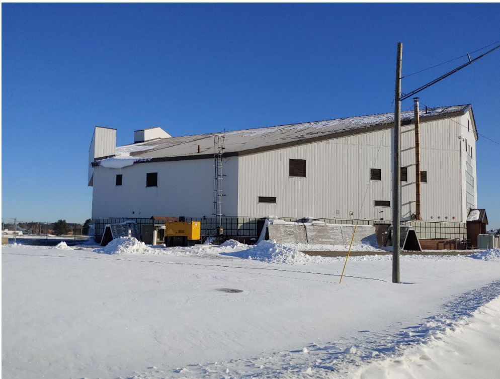
Project 8. Demolish B542 (FKNN252001): Side view of B542, looking east. (Photo credit: L. Rivard, Tetra Tech, 1/11/2021.)
