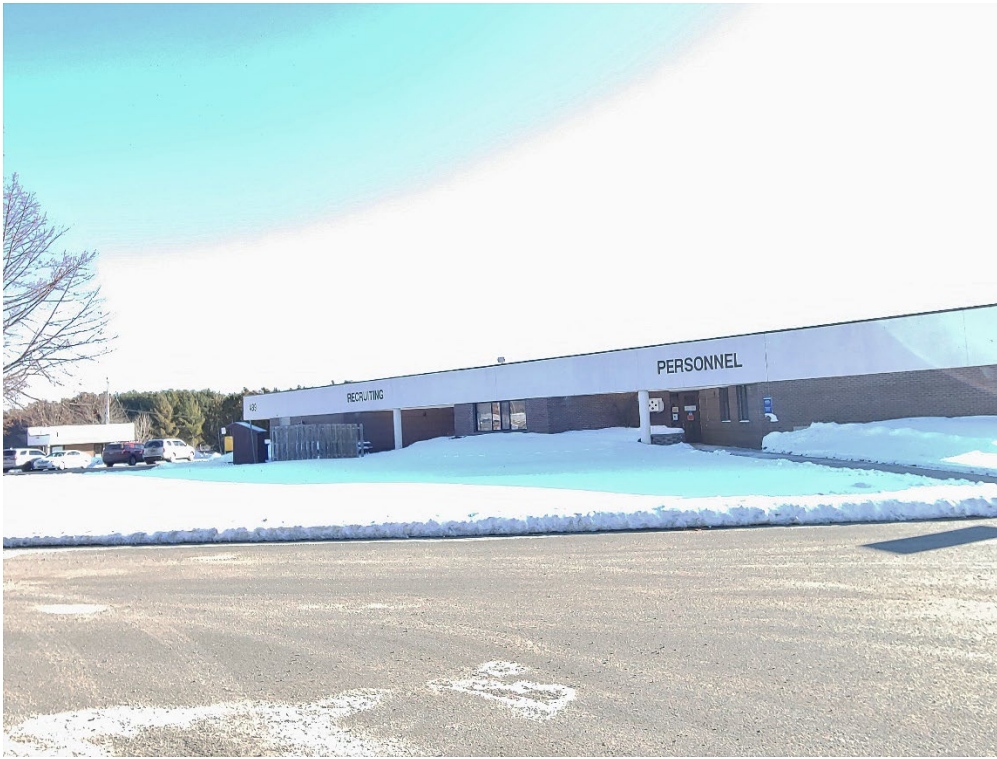
Project 6. Demolish B489 and B505 (FKNN232003): View of B489, looking northeast. (Photo credit: L. Rivard, Tetra Tech, 1/11/2021.)
