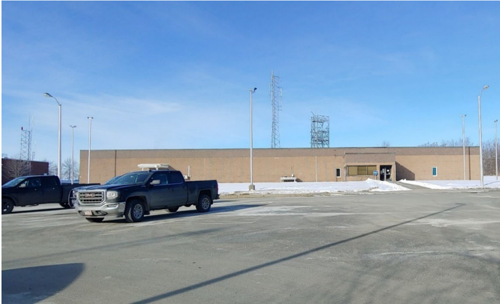
Project 4. Demolish B510 (FKNN212001): View of B510, looking northwest. (Photo credit: L. Rivard, Tetra Tech, 1/11/2021.)
