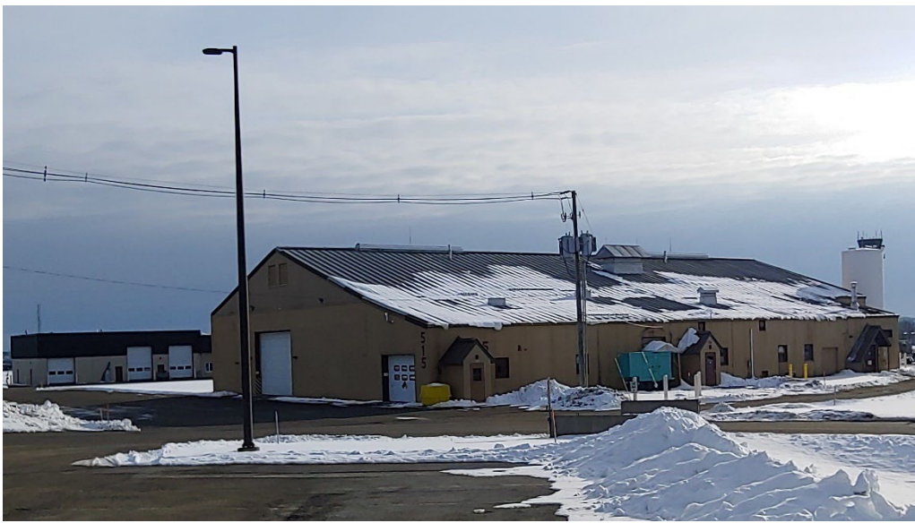
Project 5. Interior renovations to B515 for SAT (FKNN212002): View of B515, looking southeast. (Photo credit: L. Rivard, Tetra Tech, 1/11/2021.)
