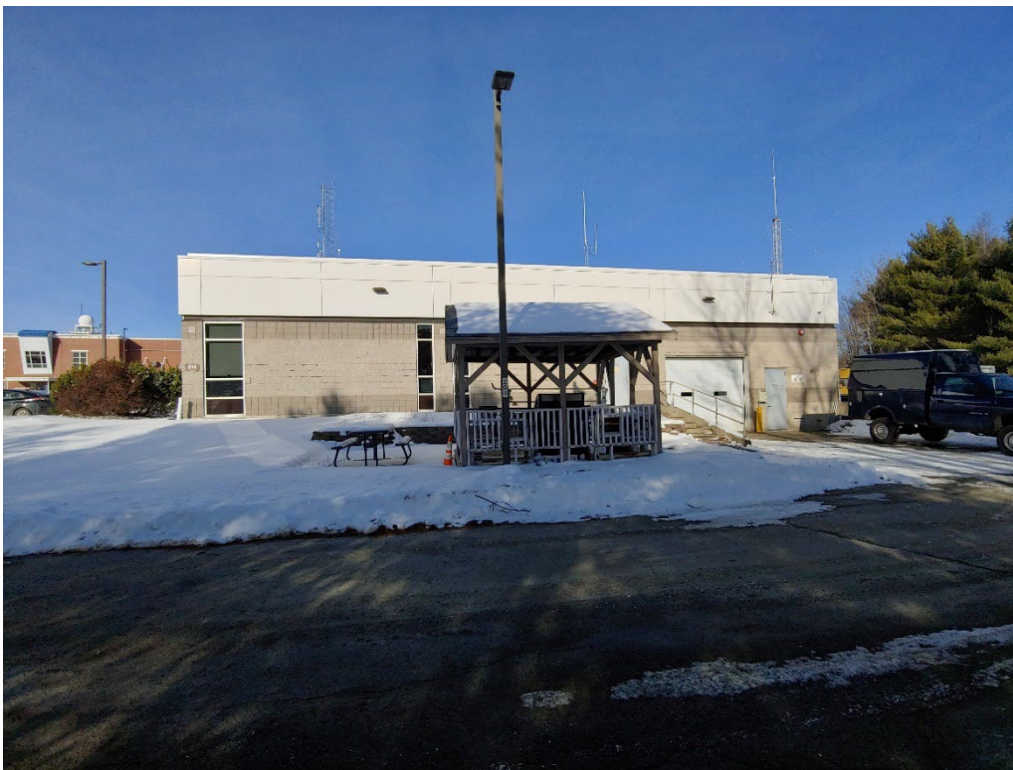
Project 7. ADAL to B514 (FKNN192001): B514, looking northwest. View of southeast side of B514 where proposed addition would be constructed. (Photo credit: L. Rivard, Tetra Tech, 1/11/2021.)
