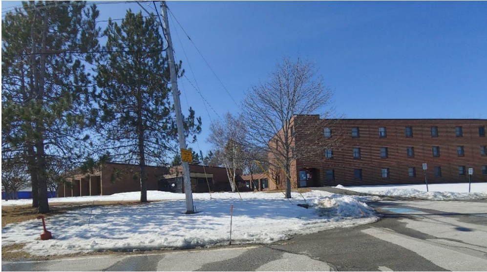
Project 10. ADAL to B417: View of B417, looking west. Dining facility (one story) on left, barracks (3 stories) on right. (Photo credit: L. Rivard, Tetra Tech, 3/10/2021.)
