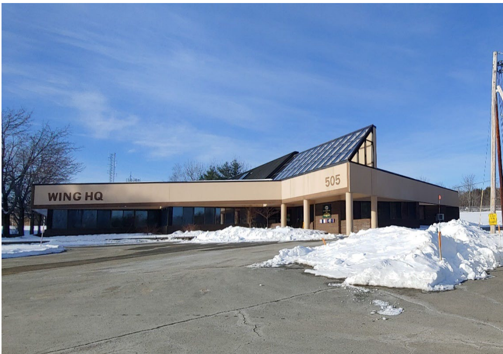
Project 6. Demolish B489 and B505 (FKNN232003): View of B505, looking west. (Photo credit: L. Rivard, Tetra Tech, 1/11/2021.)
