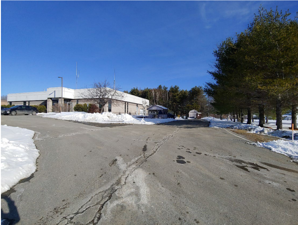
Project 7. ADAL to B514 (FKNN192001): View of B514, looking north/northeast. (Photo credit: L. Rivard, Tetra Tech, 1/11/2021.)
